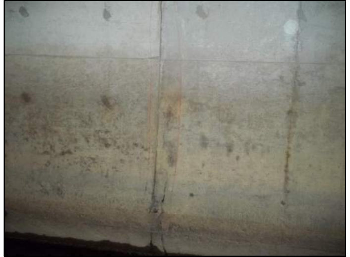
66' – Rt side Separation at joint
