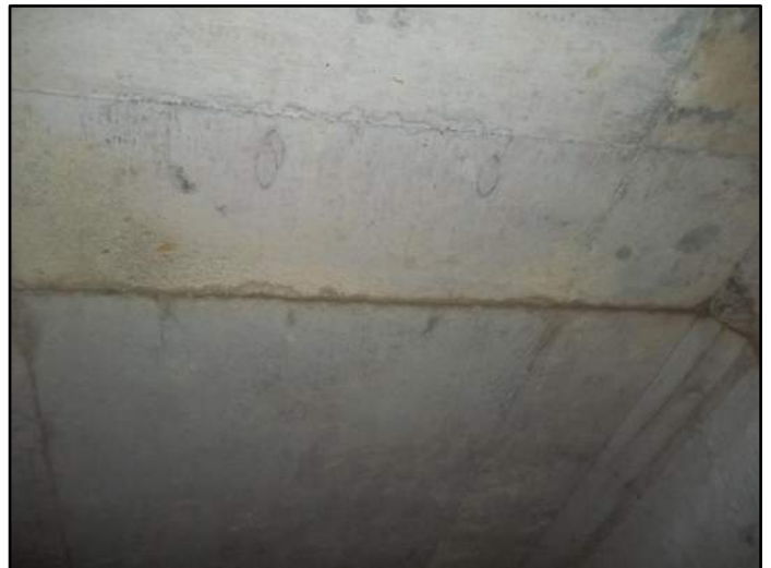
66' – Top Separation at joint
