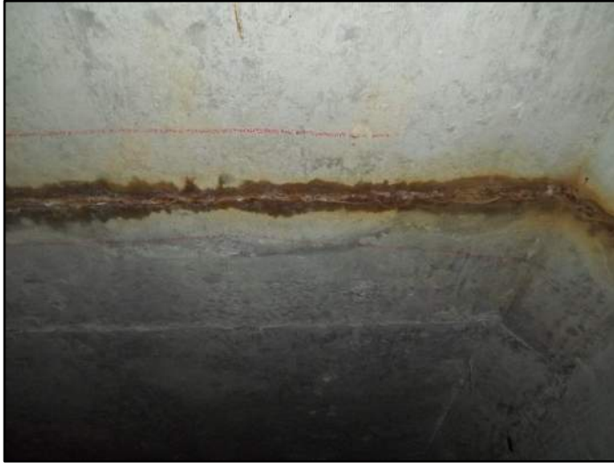
200' – Top side Transverse cracking
