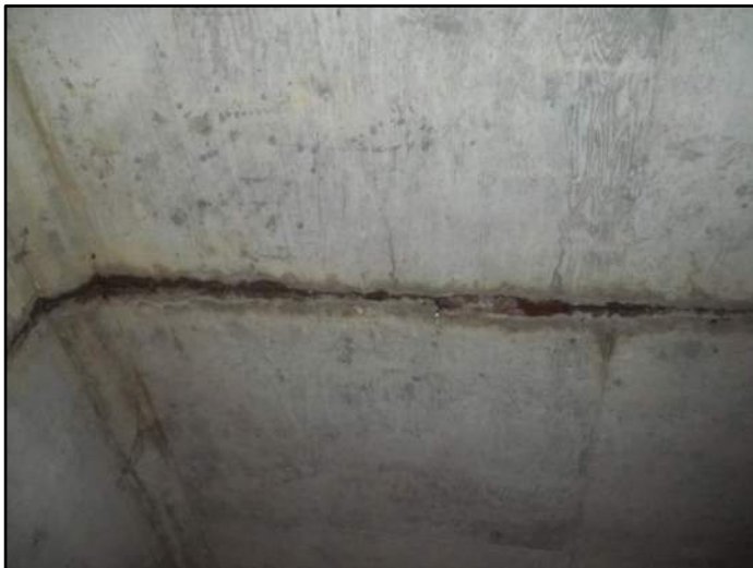
125' – Top Separation at joint
