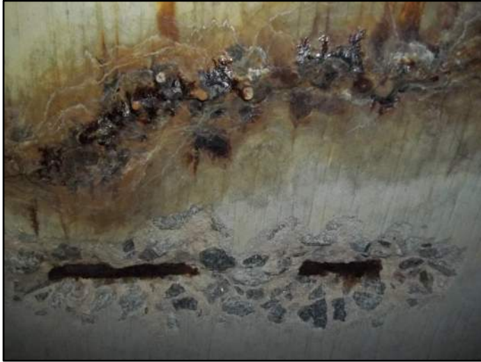
163' – Top Transverse cracking crack and exposed rebar
