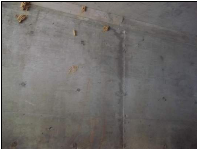
30' – Lt side Transverse Cracking
