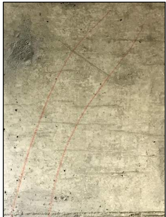
50' – Lt side Transverse cracking
