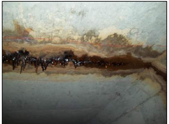
259' – Top Separation at joint
