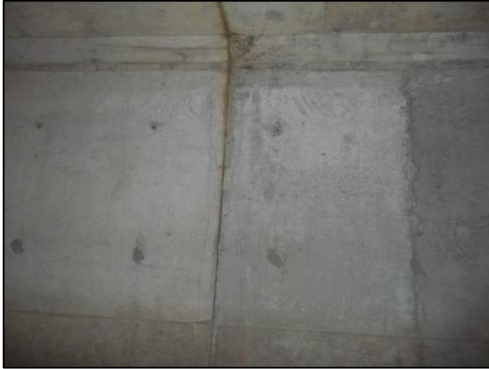
66' – Rt side Separation at joint
