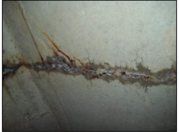
114' – Top side Transverse cracking
