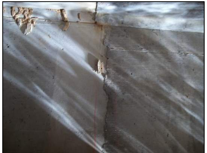
15' – Rt side Transverse Cracking
