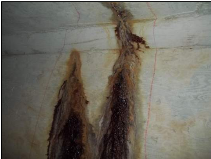
163' – Rt side Transverse cracking
