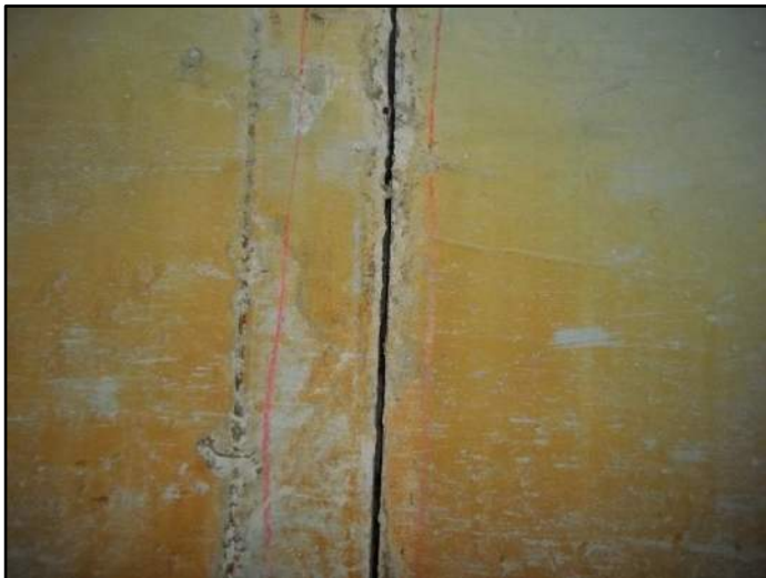
79.5' – Rt side Separation at joint
