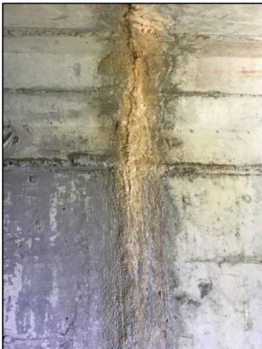
73' – Rt side Transverse cracking
