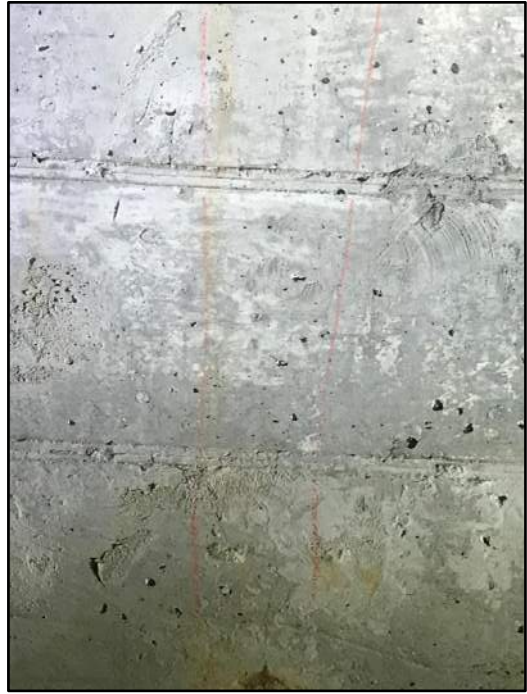
78' – Rt side Transverse cracking
