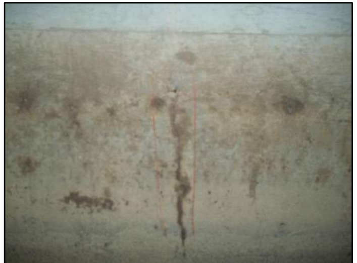
91' – Rt side Transverse Cracking with exposed rebar
