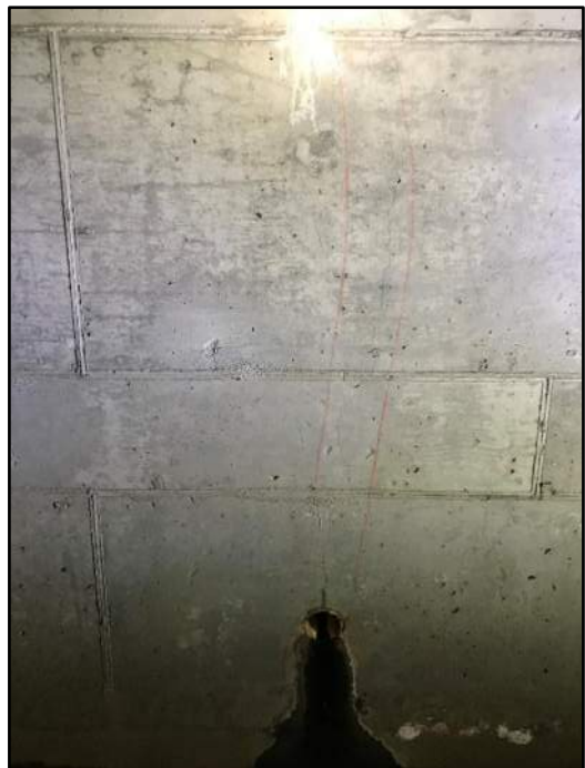
50' – Rt side Transverse cracking
