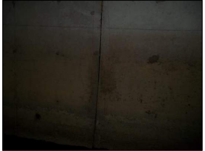
125' – Rt side Separation at joint
