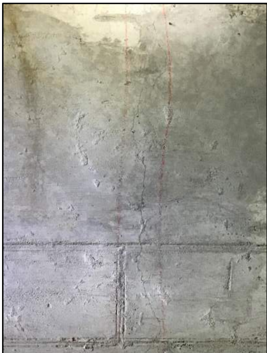
50' – Rt side Transverse cracking
