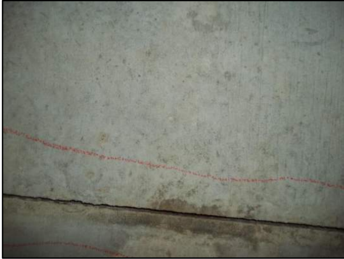
79.5' – Top Separation at joint
