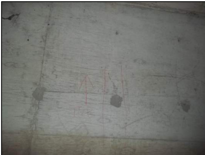
97' – Lt side Transverse Cracking
