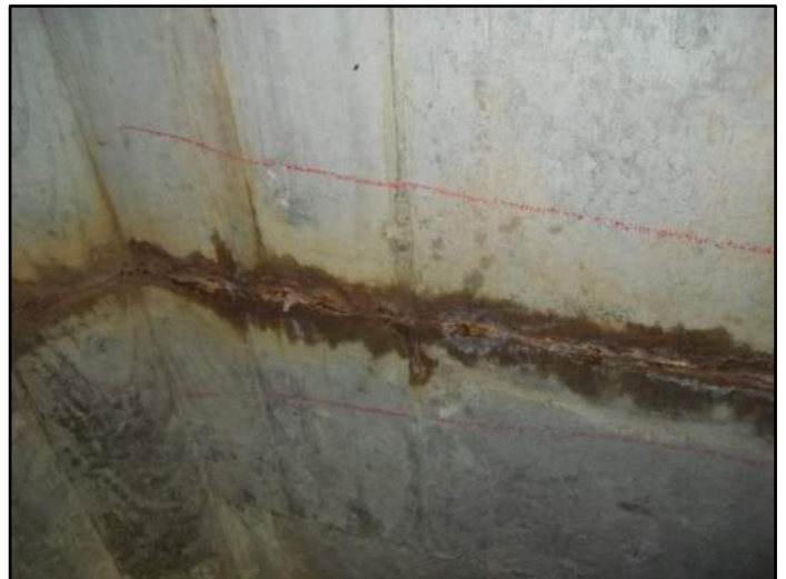
200' – Top side Transverse cracking
