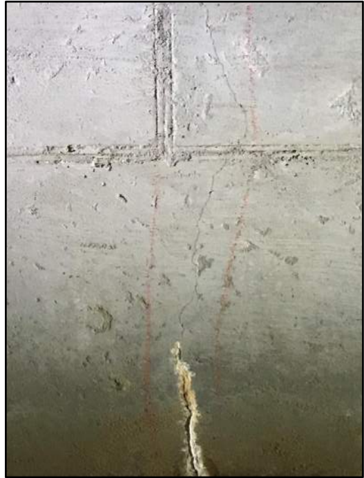
50' – Rt side Transverse cracking
