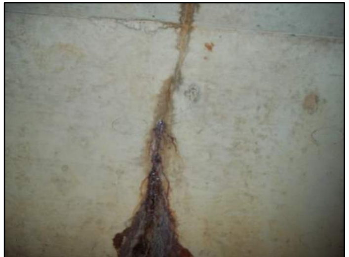
114' – Rt side Transverse cracking
