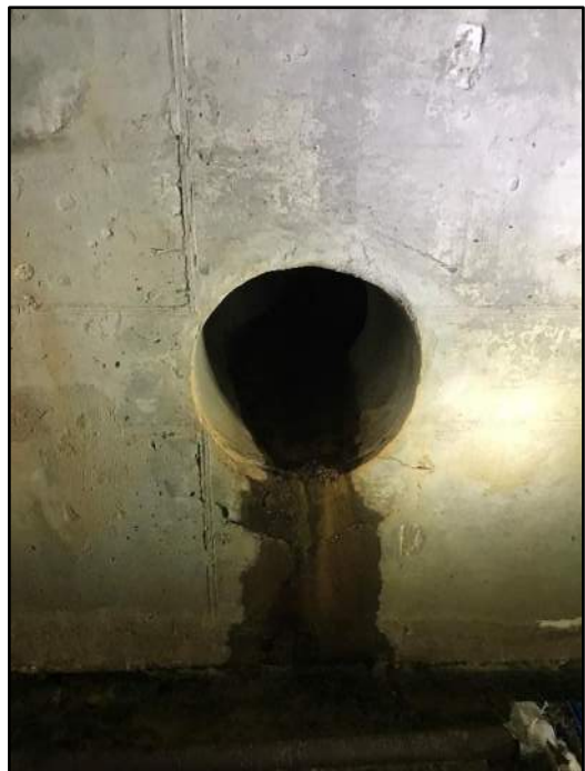
85' – Rt side 18" RCP cracking at tie interface
