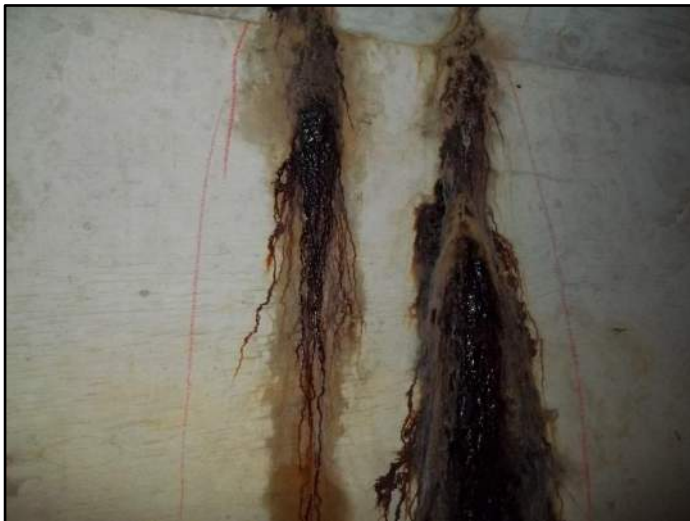
163' – Lt side Transverse cracking
