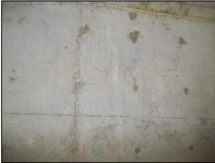
146' – Lt side Transverse Cracking
