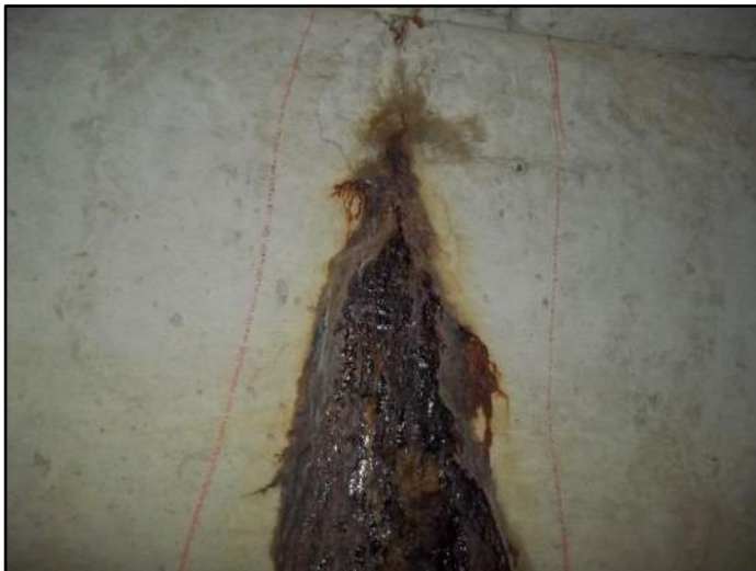
98' – Lt side and top Transverse cracking
