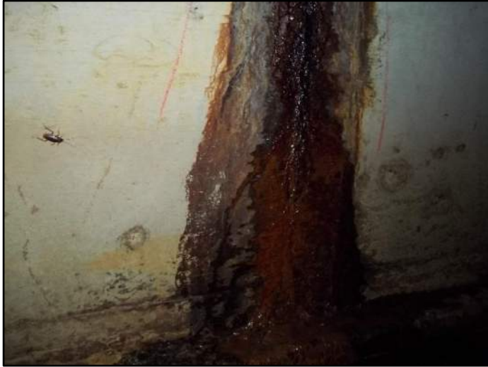
200' – Lt side Transverse cracking
