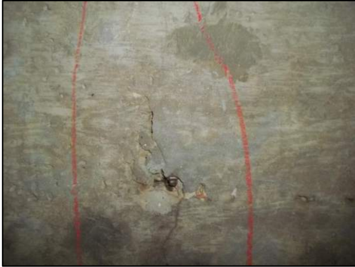
91' – Rt side Transverse Cracking with exposed rebar
