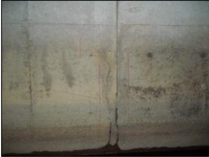
66' – Lt side Separation at joint
