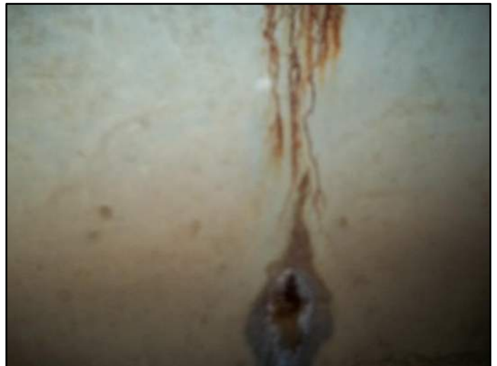
114' – Lt side Transverse cracking
