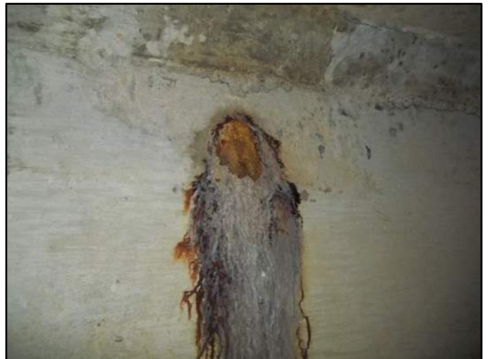
228' – Lt side Weeping crack
