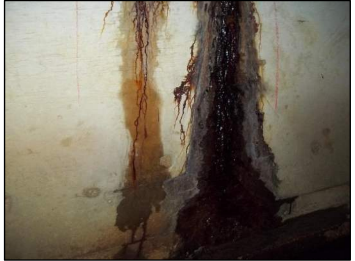
163' – Lt side Transverse cracking
