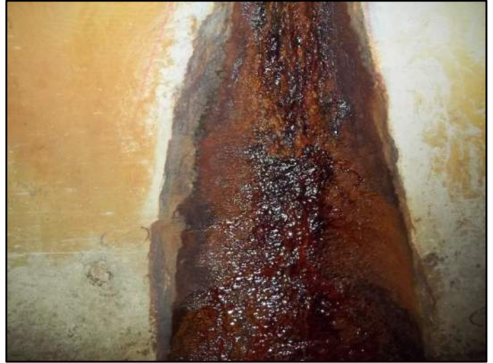
139.5' – Lt side Separation at joint
