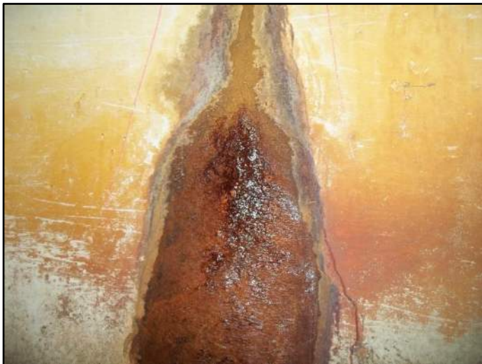
139.5' – Rt side Separation at joint
