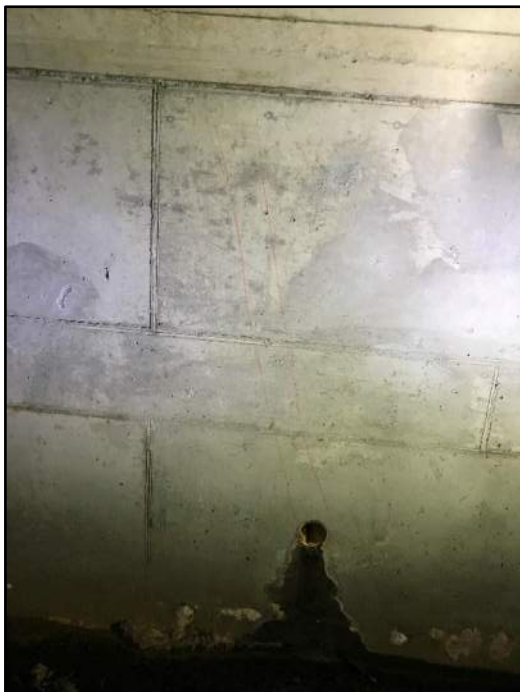
63' – Rt side Transverse cracking
