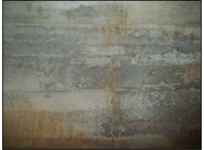
32' – Rt side Transverse cracking
