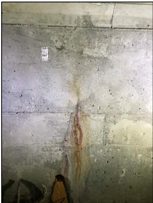
95' – Rt side Transverse cracking
