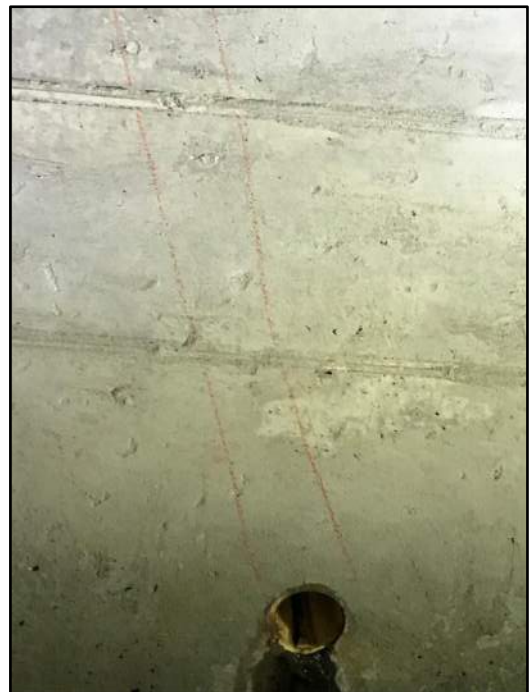
63' – Rt side Transverse cracking
