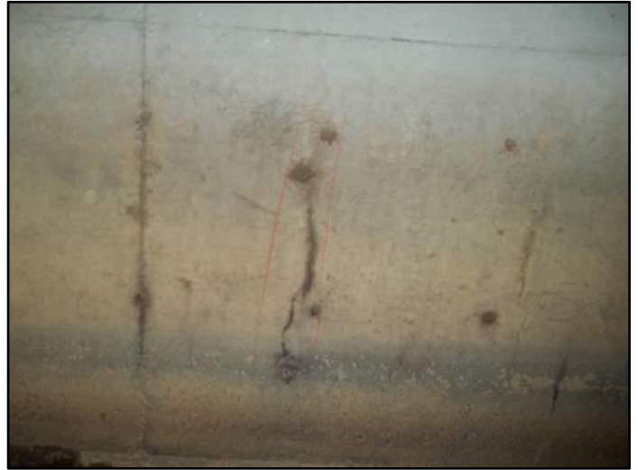
146' – Rt side Transverse Cracking
