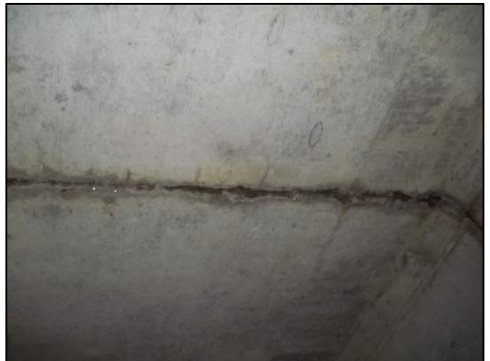
125' – Top Separation at joint
