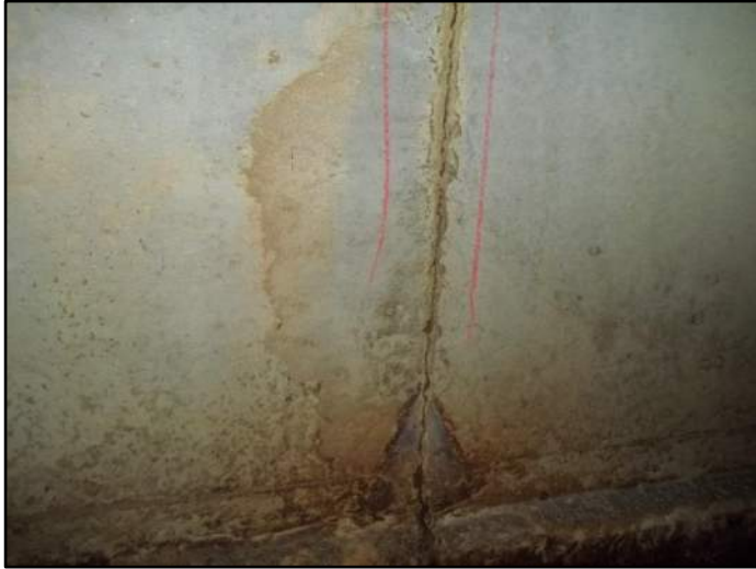
259' – Lt side Separation at joint
