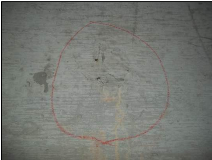
115' – Rt side Exposed rebar
