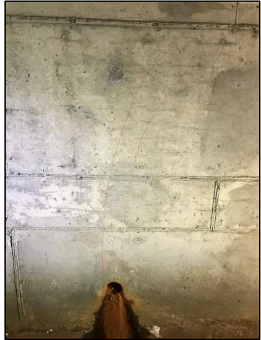
50' – Lt side Transverse cracking
