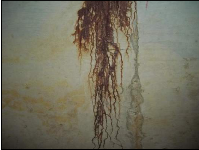
143' – Rt side weeping crack
