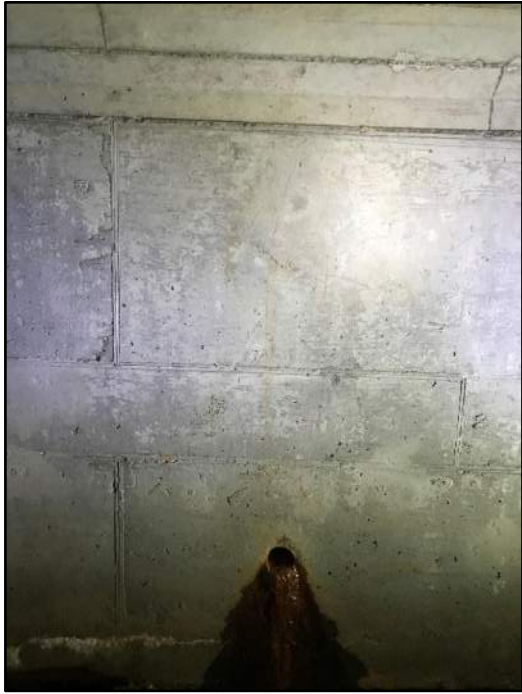
78' – Rt side Transverse cracking
