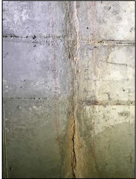
69' – Rt side Transverse cracking
