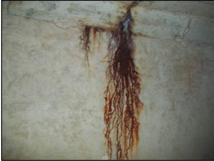
114' – Lt side Transverse cracking
