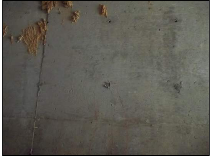
40' – Rt side Transverse Cracking
