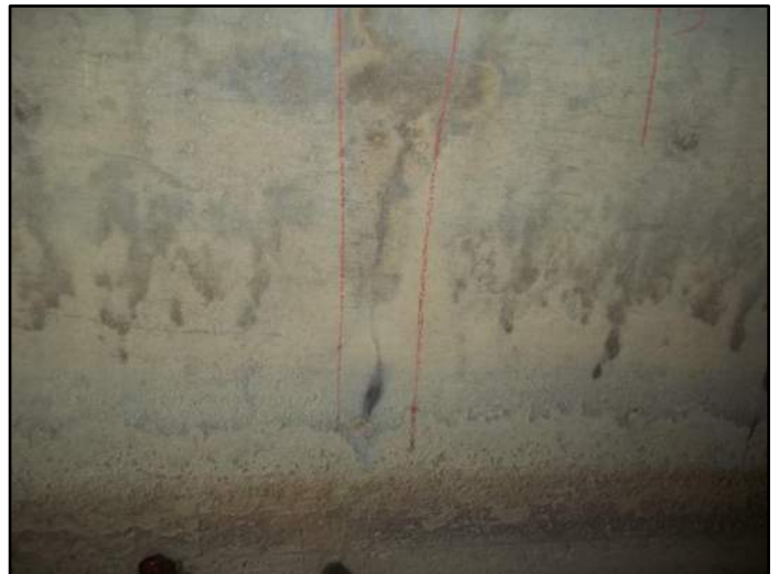
43' – Lt side Transverse Cracking
