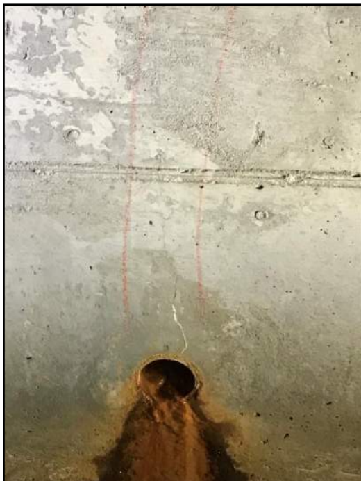
50' – Lt side Transverse cracking
