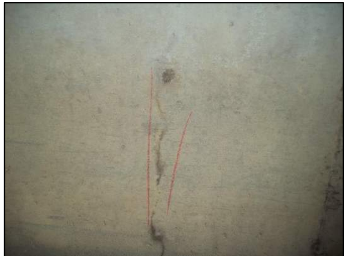
139' – Rt side Transverse Cracking
