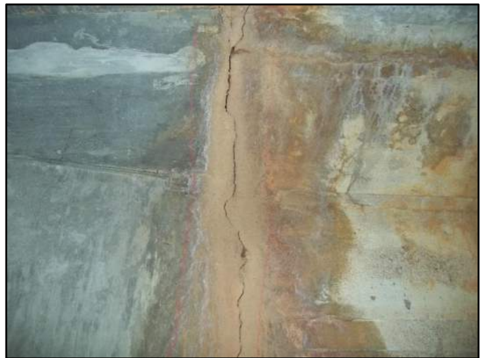
136' – Lt side Transverse cracking
