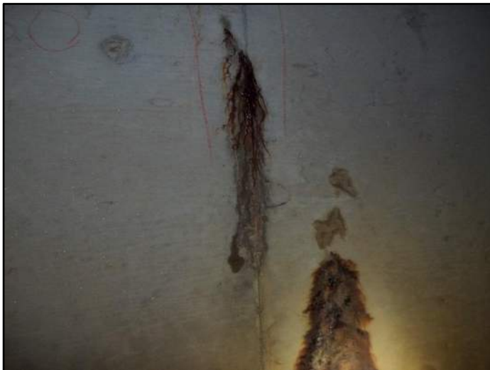
100' – Rt side Transverse cracking
