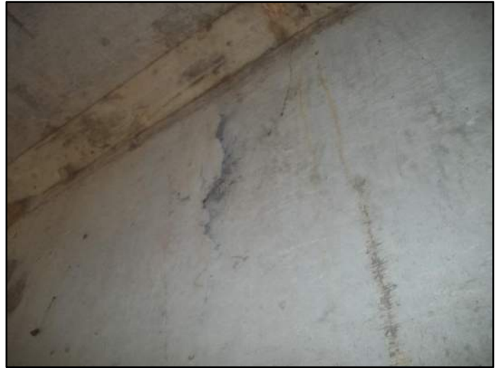
151' – Rt side Spalling at top corner
