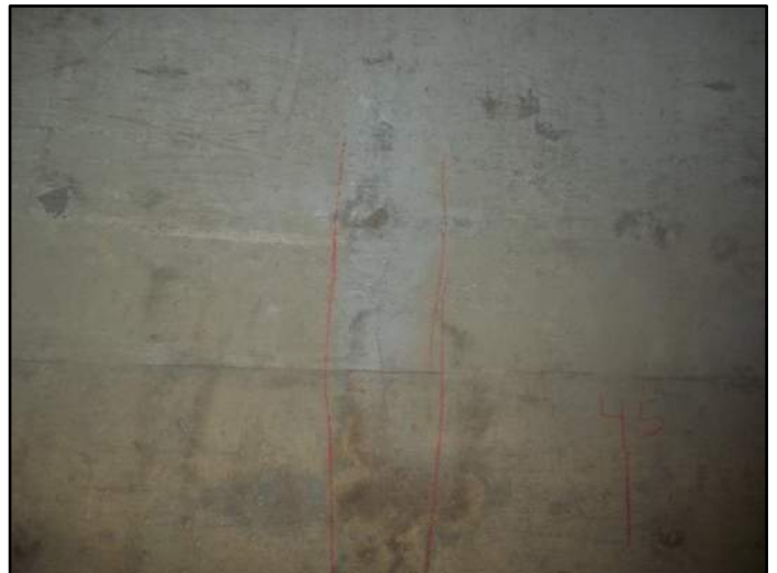
43' – Lt side Transverse Cracking
