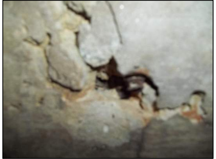
91' – Rt side Transverse Cracking with exposed rebar
