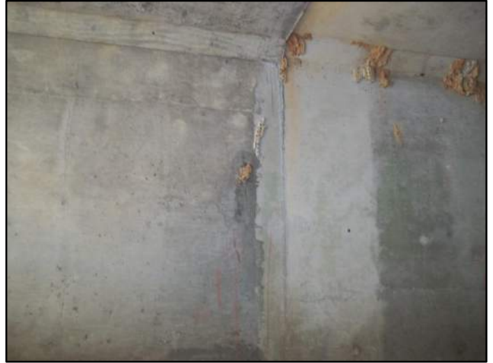
15' – Lt side Transverse Cracking
