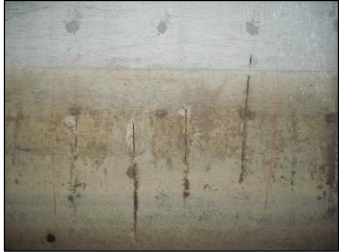
98 – 102' – Rt side Exposed rebar
