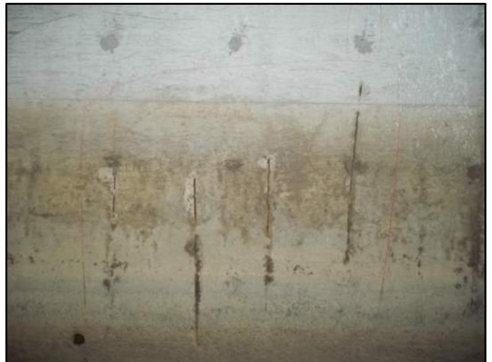
98 – 102' – Rt side Exposed rebar
