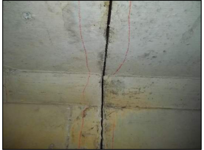
79.5' – Top Separation at joint
