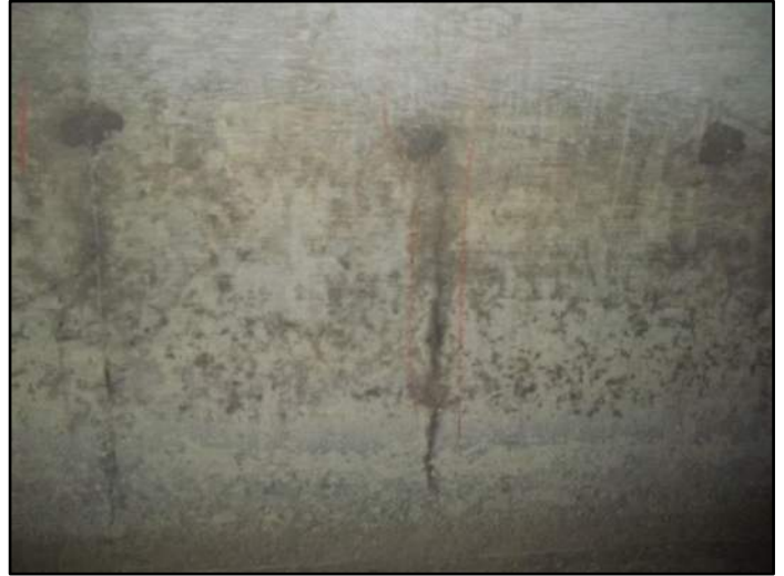
97' – Lt side Vertical crack
