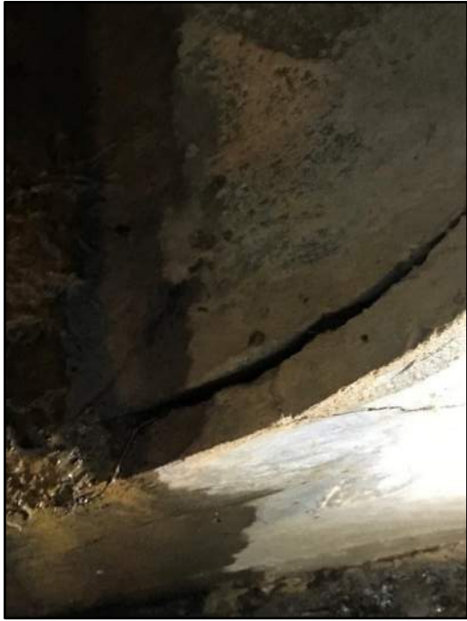
85' – Rt side 18" RCP cracking at tie interface
