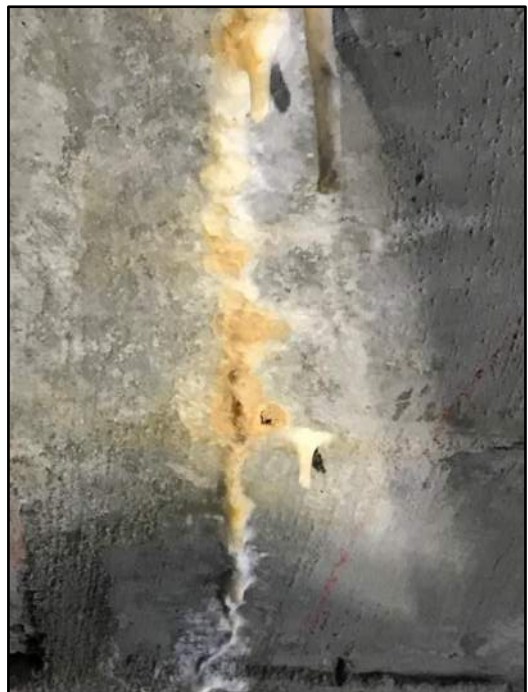
73' – Rt side Transverse cracking
