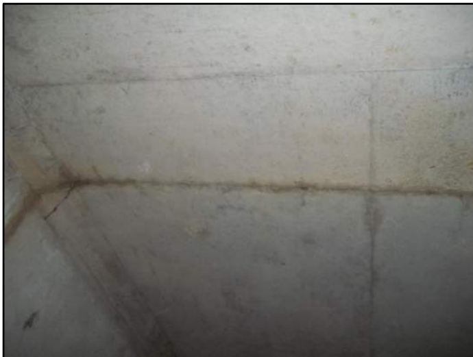
66' – Top Separation at joint
