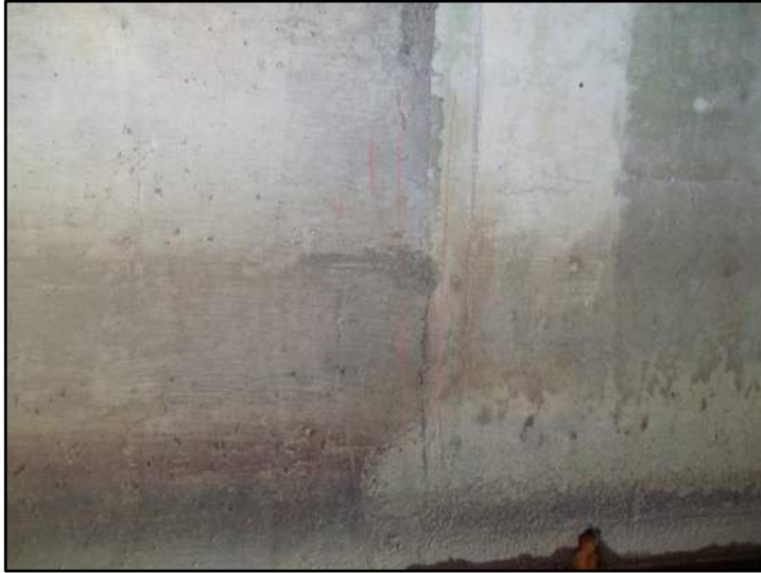
15' – Lt side Transverse Cracking
