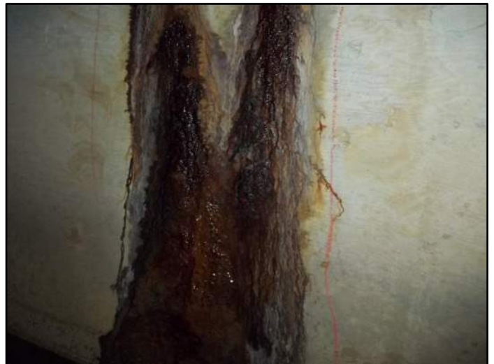
163' – Rt side Transverse cracking
