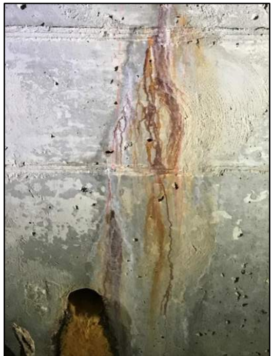
95' – Rt side Transverse cracking
