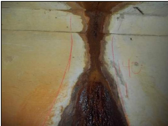
139.5' – Lt side Separation at joint
