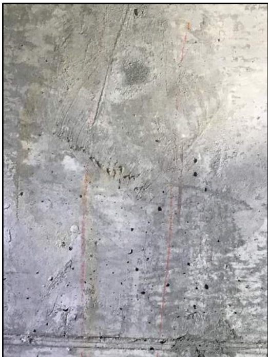
78' – Rt side Transverse cracking
