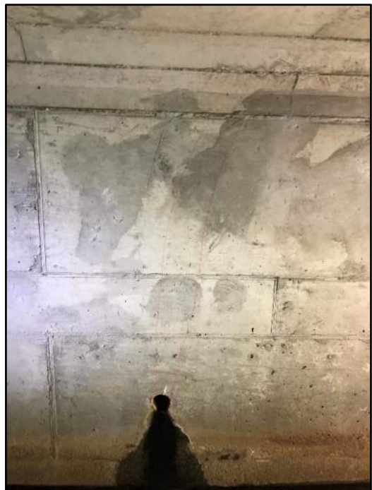
44' – Rt side Transverse cracking
