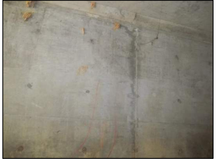
30' – Lt side Transverse Cracking
