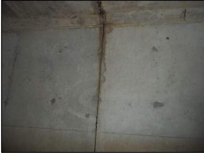
125' – Rt side Separation at joint
