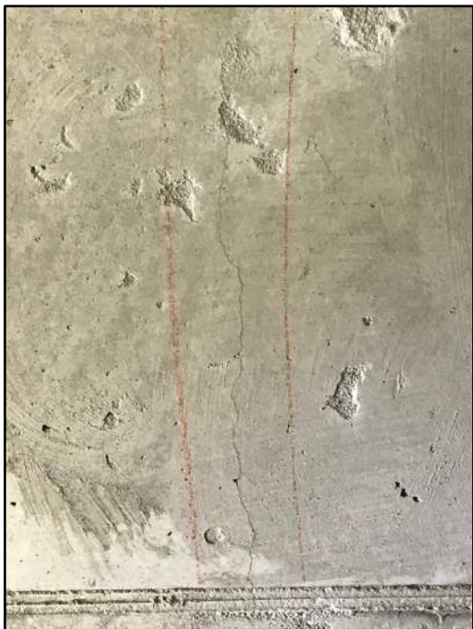
44' – Lt side Transverse cracking
