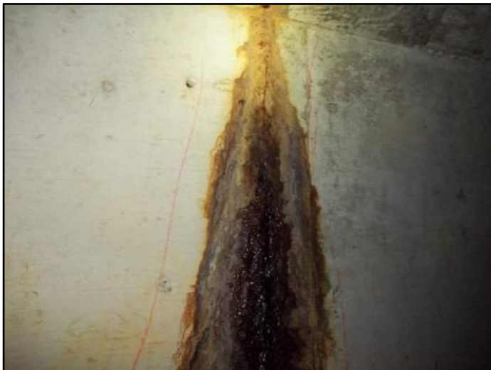
200' – Lt side Transverse cracking
