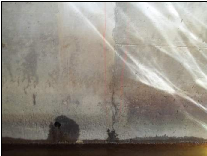
15' – Rt side Transverse Cracking
