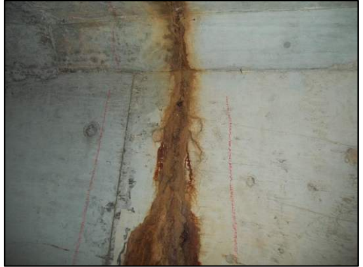
200' – Rt side Transverse cracking
