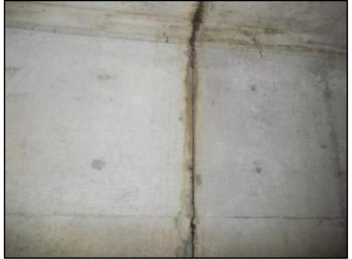
125' – Lt side Separation at joint
