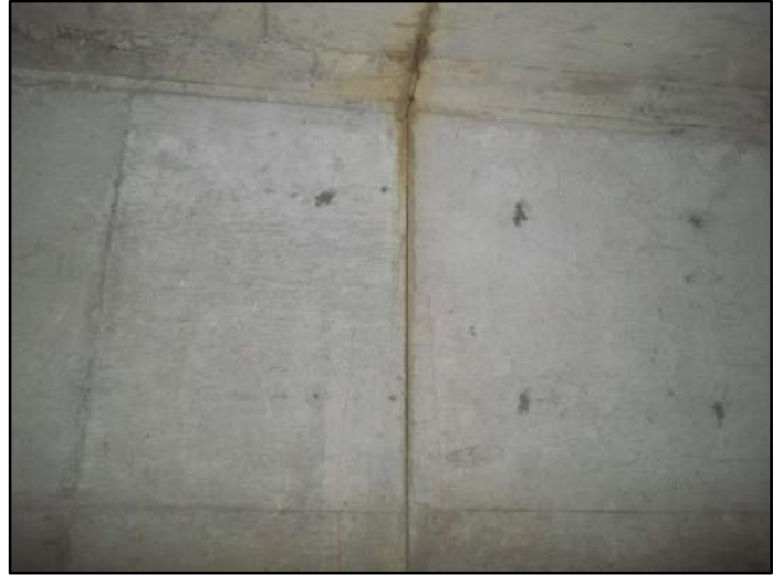
66' – Lt side Separation at joint
