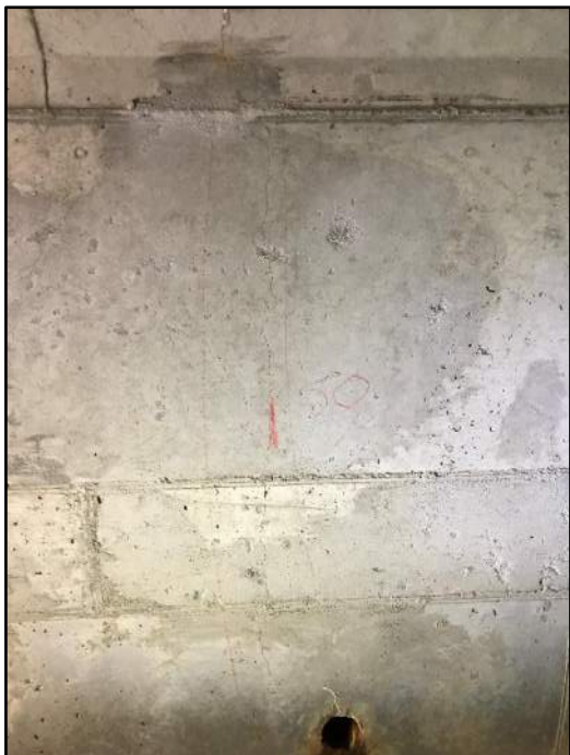
44' – Rt side Transverse cracking
