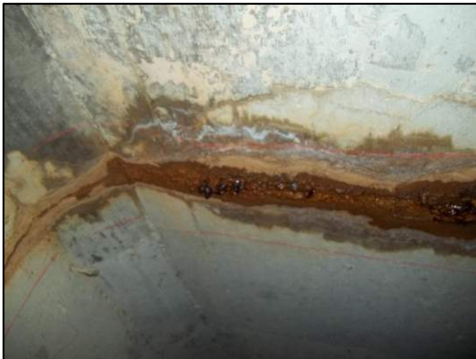
259' – Top Separation at joint
