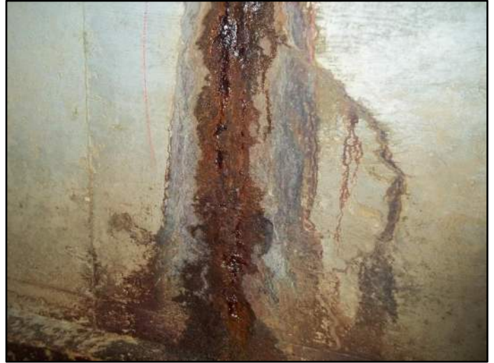
259' – Rt side Separation at joint
