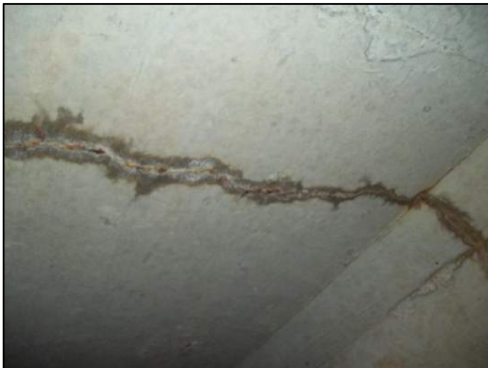
114' – Top side Transverse cracking
