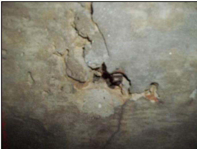
91' – Rt side Transverse Cracking with exposed rebar
