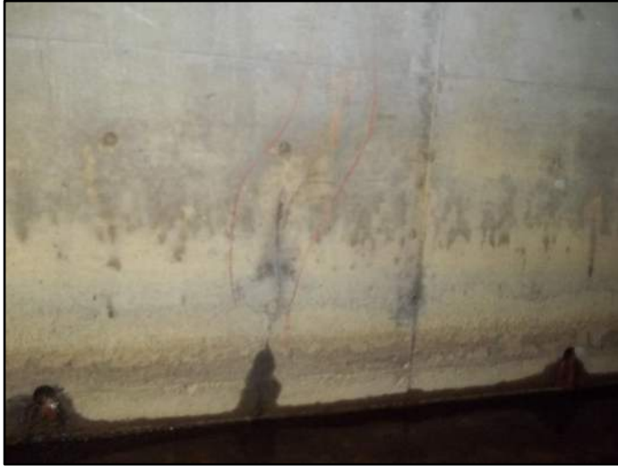
30' – Lt side Transverse Cracking
