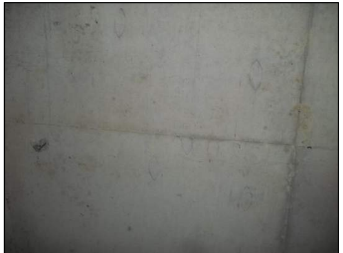
97' – Top Transverse Cracking
