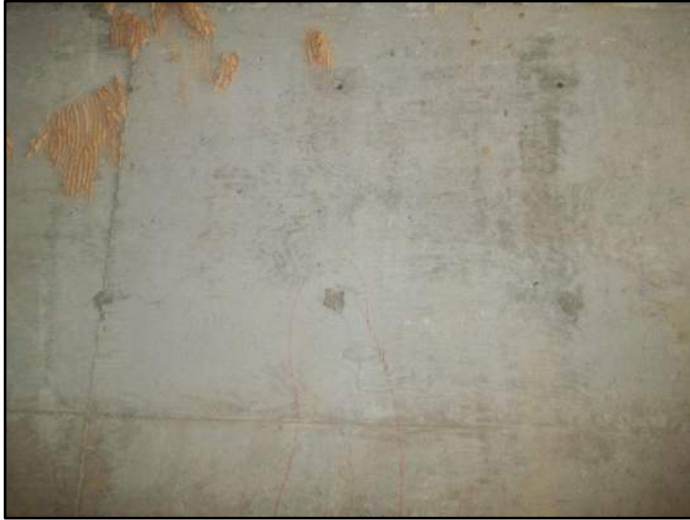
30' – Rt side Transverse Cracking
