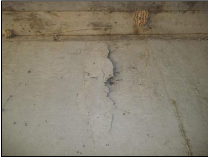
151' – Rt side Spalling at top corner
