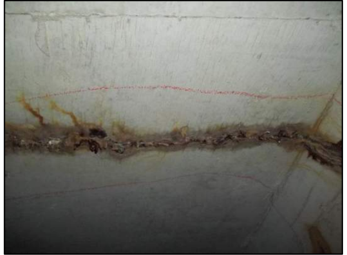
163' – Top side Transverse cracking
