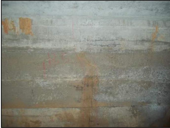
23' – Lt side Transverse cracking
