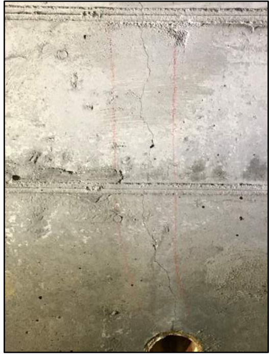
44' – Lt side Transverse cracking
