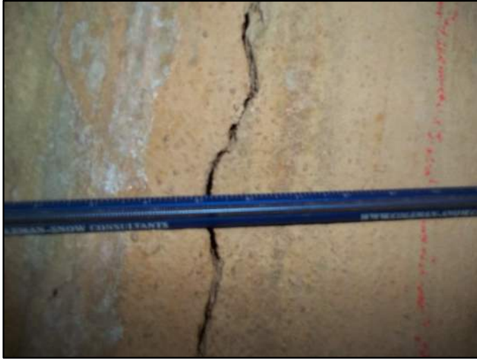
136' – Lt side Transverse cracking
