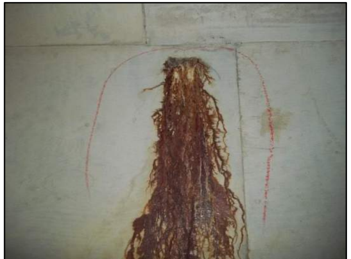
143' – Rt side weeping crack
