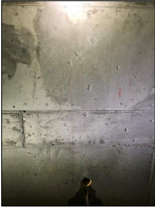
44' – Lt side Transverse cracking
