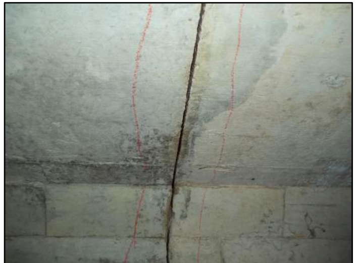
79.5' – Lt side Separation at joint
