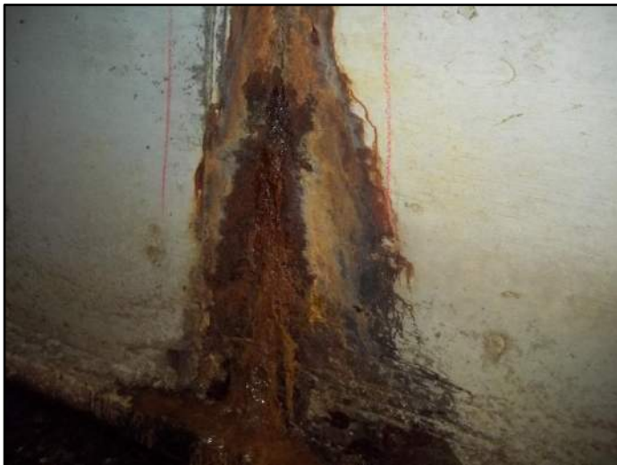
200' – Rt side Transverse cracking
