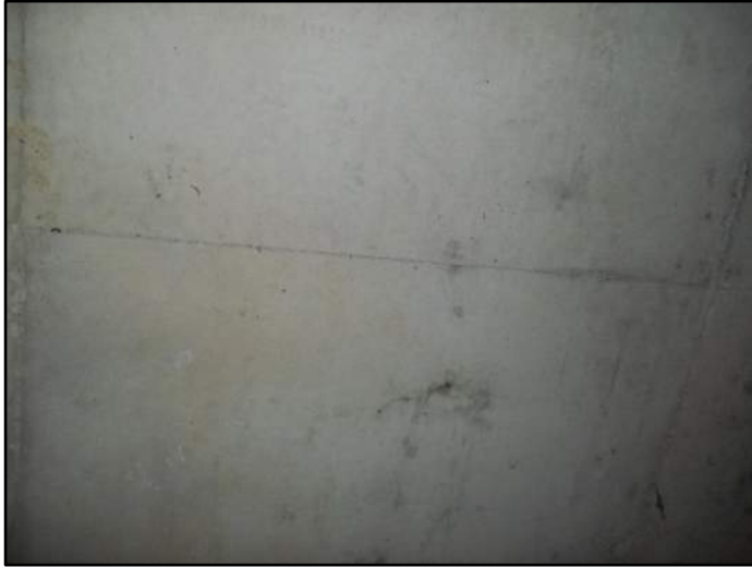
97' – Top Transverse Cracking
