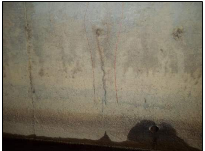
30' – Rt side Transverse Cracking
