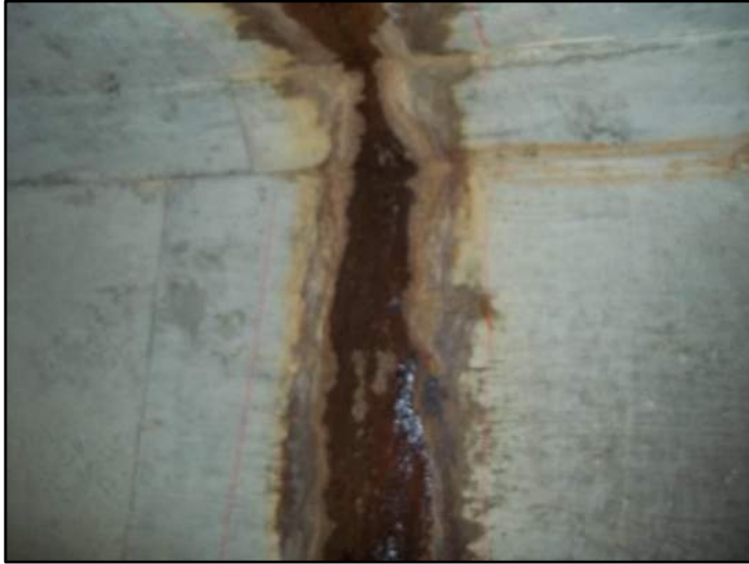
259' – Rt side Separation at joint
