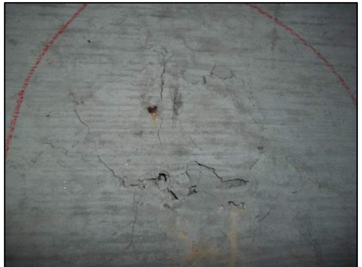
115' – Rt side Exposed rebar
