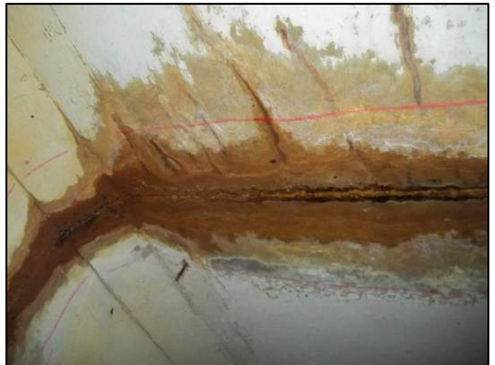
139.5' – Top side Separation at joint
