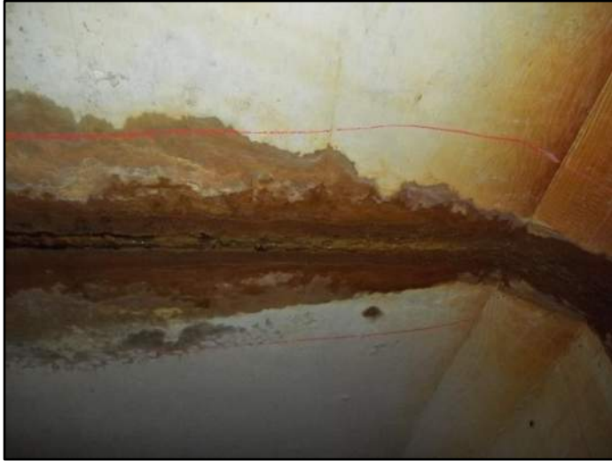
139.5' – Top side Separation at joint
