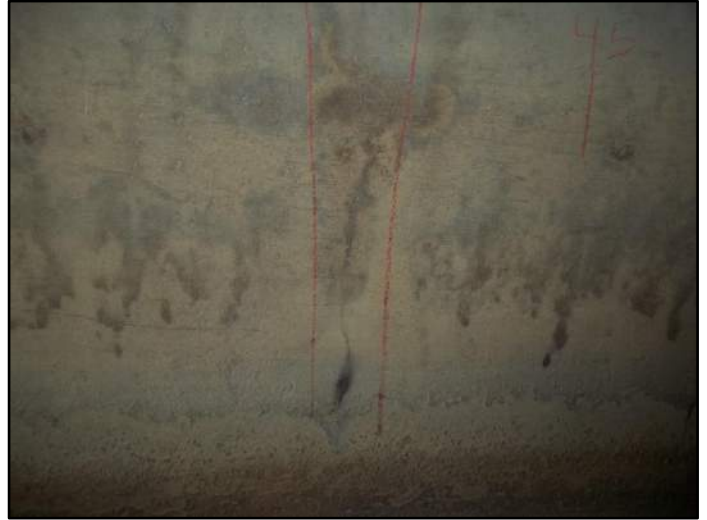
43' – Lt side Transverse Cracking
