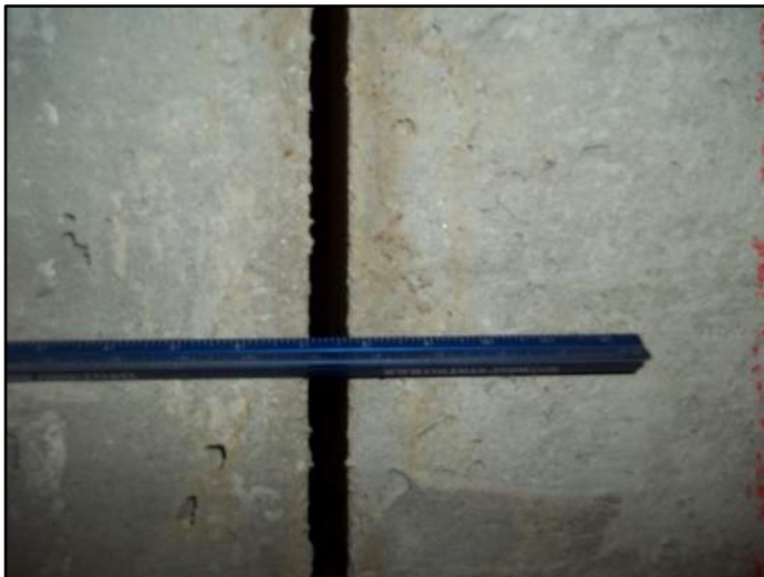
66' – Lt side Separation at joint
