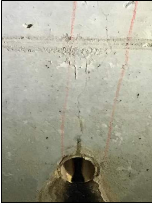
55' – Rt side Transverse cracking
