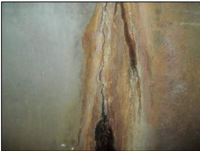
113' – Lt side Transverse cracking
