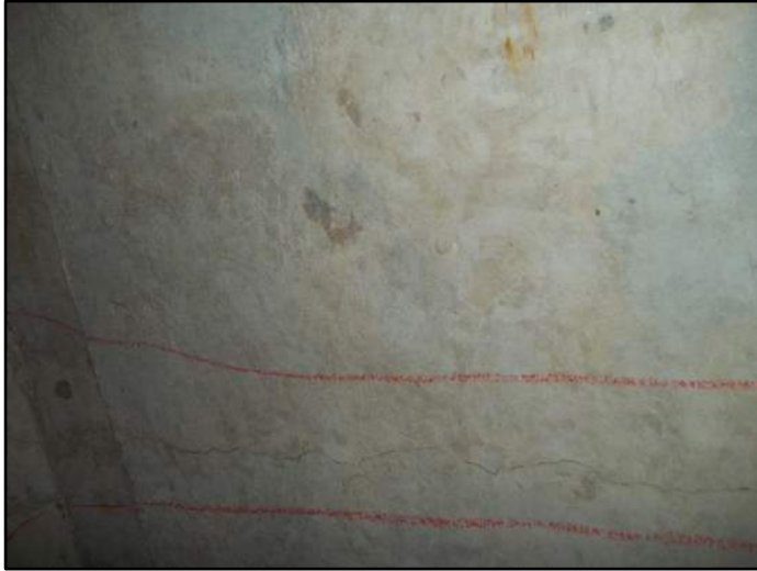
98' – Lt side and top Transverse cracking
