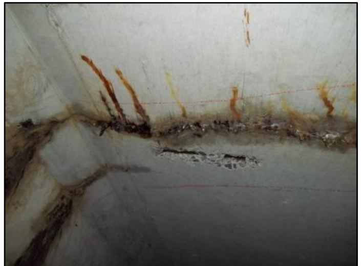
163' – Top Transverse cracking with exposed rebar
