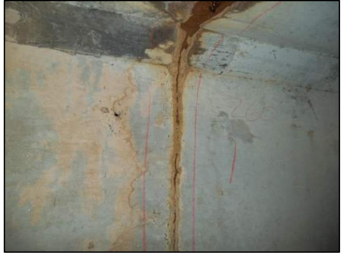
259' – Lt side Separation at joint
