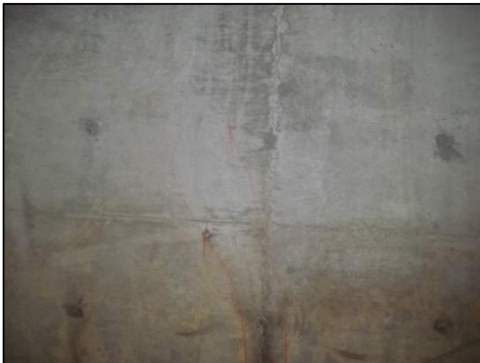
40' – Rt side Transverse Cracking
