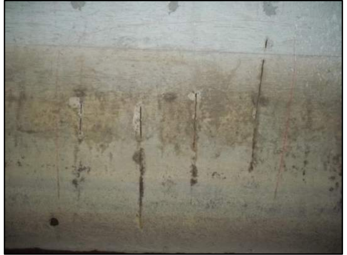
98 – 102' – Rt side Exposed rebar
