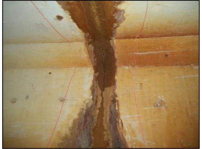
139.5' – Rt side Separation at joint
