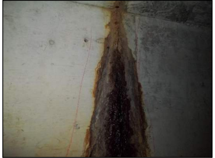
200' – Lt side Transverse cracking
