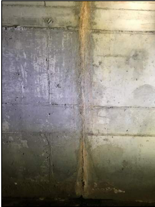
69' – Rt side Transverse cracking
