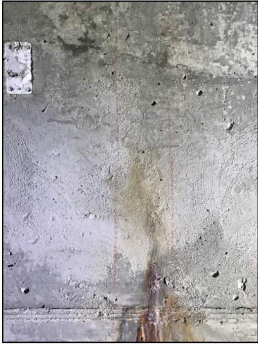
110' – Rt side Transverse cracking
