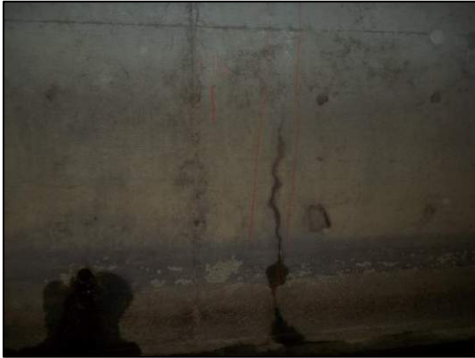
146' – Lt side Transverse Cracking
