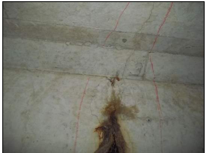
98' – Lt side and top Transverse cracking
