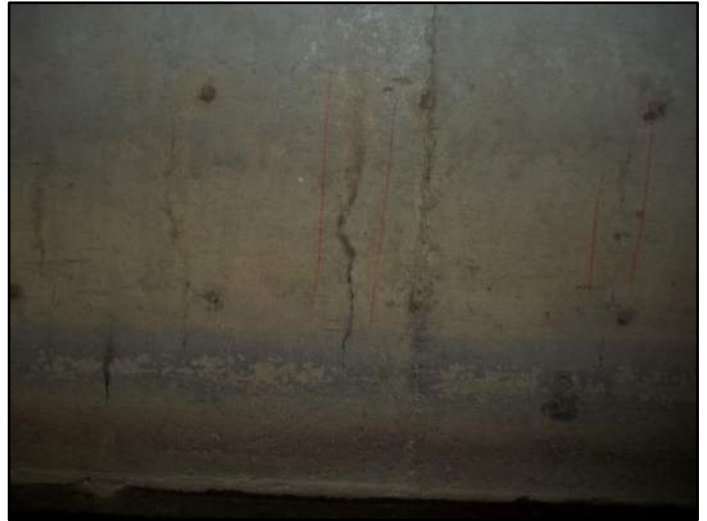
146' – Rt side Transverse Cracking
