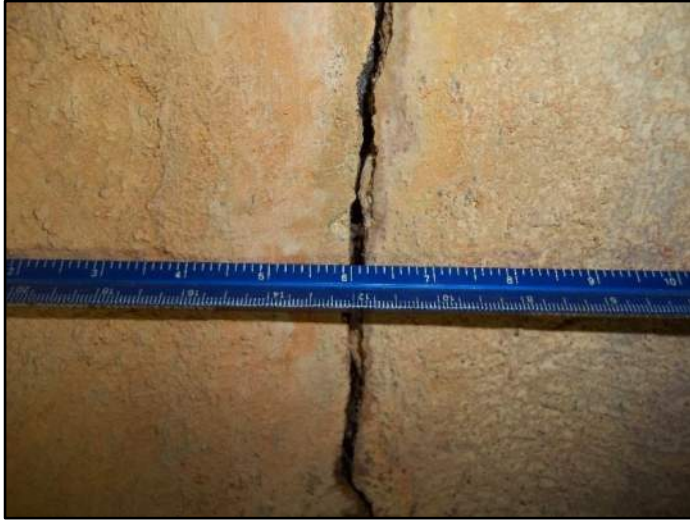
79.5' – Lt side Separation at joint
