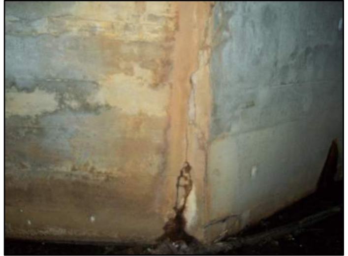
140' – Rt side Transverse cracking
