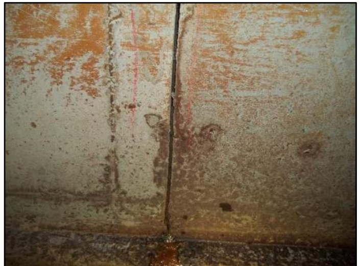
79.5' – Rt side Separation at joint
