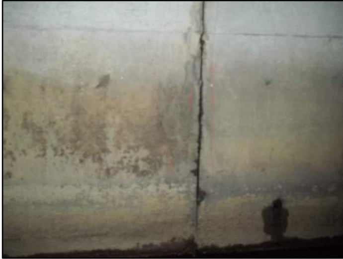
125' – Lt side Separation at joint
